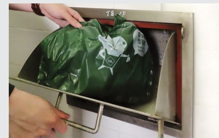
Inlet of refuse chute on individual floor
