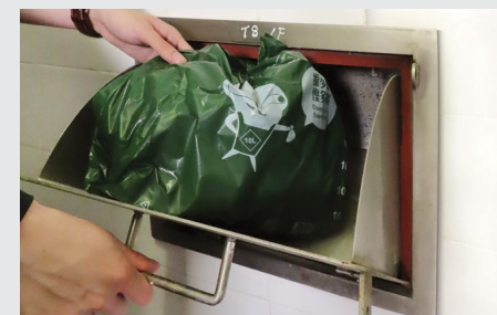
Inlet of refuse chute on individual floor
