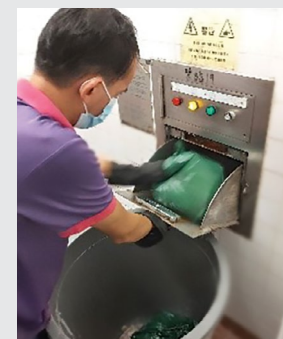
Refuse chute inlets that are linked to ARCSs
