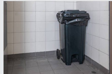
Refuse rooms on individual floor
