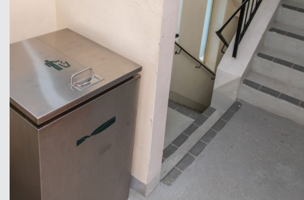
Waste collection bin at staircase landing (i)
