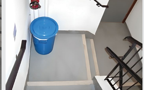
Waste collection bin at staircase landing (ii)
