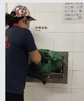
Refuse chute inlets
