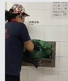
Refuse chute inlets
