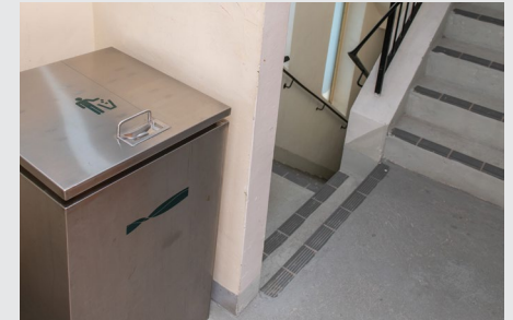
Waste collection bin at staircase landing
