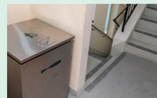
Waste collection bin at the staircase landing
