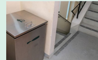
Waste collection bin at the staircase landing
