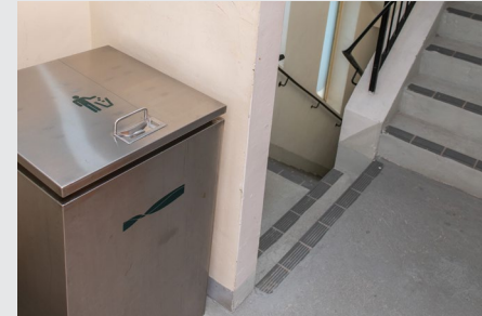
Waste collection bin at staircase landing (i)
