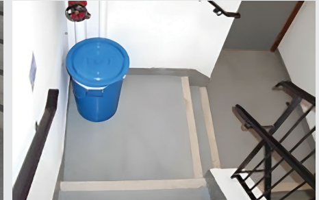
Waste collection bin at staircase landing (ii)
