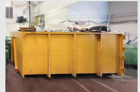
Oversized waste reception areas (ii)
