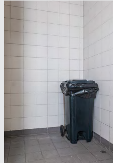
Refuse rooms on individual floor
