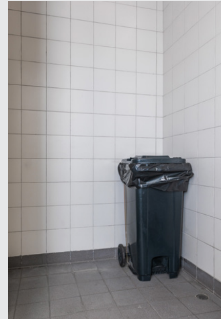
Refuse rooms on individual floor
