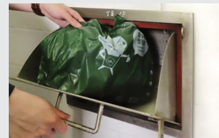
Inlet of refuse chute on individual floor
