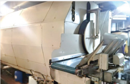
The fixed compactor is installed inside the refuse room. Waste can be discharged onto a RCV for onward delivery after compaction
