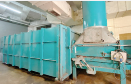
The system uses underground suction pipes to convey waste that is deposited into the refuse chute inlets on individual floors to the centrifugal chamber at the central refuse collection station. The waste will be collected for onward delivery after compaction
