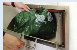
Inlet of refuse chute on individual floor
