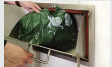
Inlet of refuse chute on individual floor
